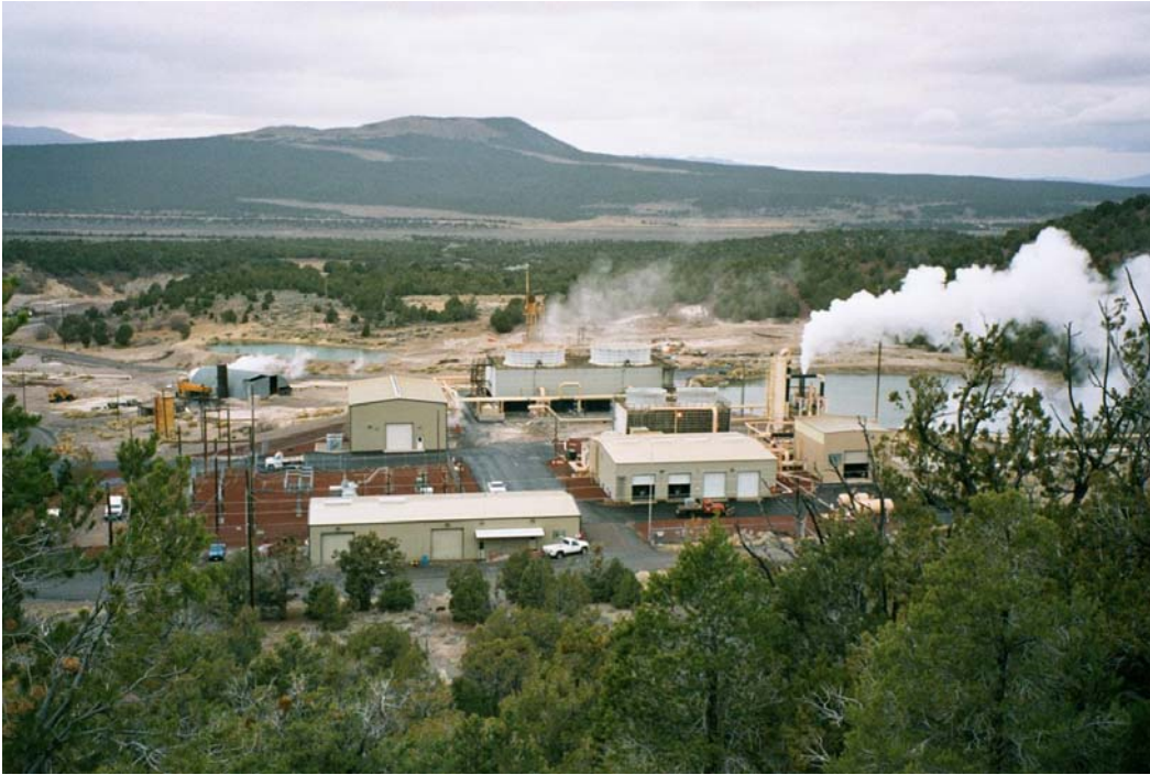
Cove Fort power facilities – Source: http://www.ampresources.com/projects.php?page=cove (used by permission)
